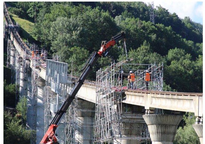
Installing an expansion device.
