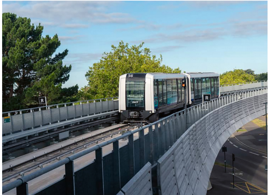
Second automatic line in Rennes: line B.
